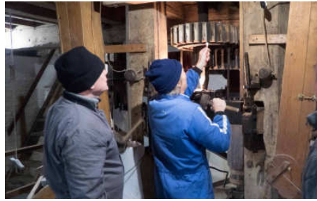
Replacing worn and broken wooden teeth in the mill's gearing
