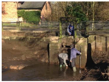
Repairing seals on the sluice to reduce water wastage.
