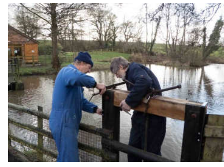
Replacing the top timber of the main mill sluice gate
