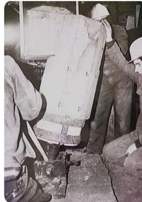
Splicing in a new section
