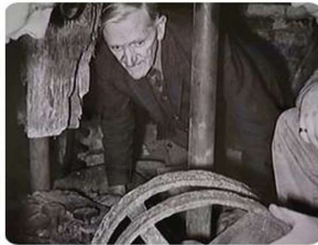
Tom Parker inspecting the broken wallower shaft.
